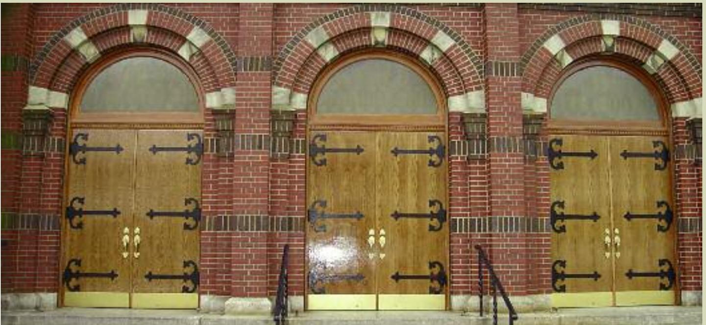
Doors were stripped, sanded, stained and varnished. Existing hardware was cleaned and polished.
