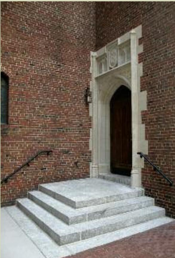
An exterior power wash, pointing, cleaning and caulking of brickwork, refinishing of wood doors and the removal and resetting of the front entrance steps complete the enhancement to the entrance to this beautiful Church. The St. Catherine of Siena statue was relocated to the priory entrance. Benches and floral planters were introduced in designated areas. All iron work was restored and painted.
