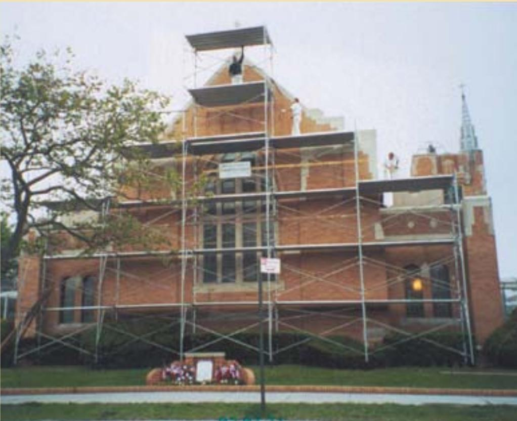
Extensive scaffold was erected and the entire masonry brick building, including limestone, cornices, sills and decorative trim received pressure washing, pointing and sealing to prevent water penetration. Flat roofs were replaced as required, window frames were re-caulked, gutters and leaders were assured proper function and the exterior doors were refinished.
